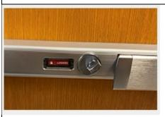
This lock includes a window which shows whether the door is locked or unlocked. In this photo, the door is locked when the thumb turn is turned to the left (counterclockwise).
