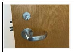
This is a standard door lock, which sits above the door handles. This lock can be used by turning the thumb turn towards the door frame to lock the door. The thumb turn can be turned away from the door frame to unlock the door.
