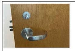
This is a standard door lock, which sits above the door handles. This lock can be used by turning the thumb turn towards the door frame to lock the door. The thumb turn can be turned away from the door frame to unlock the door.
