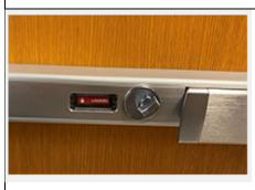
This lock includes a window which shows whether the door is locked or unlocked. In this photo, the door is locked when the thumb turn is turned to the left (counterclockwise).
