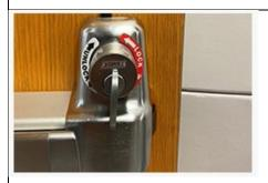
This lecture hall style lock is placed on doors with a push bar. The lock includes instructions so your which way to turn the thumb turn to ensure the door is locked. In this photo, the thumb turn would be turned counterclockwise to lock the door and would be turned clockwise to unlock the door.
