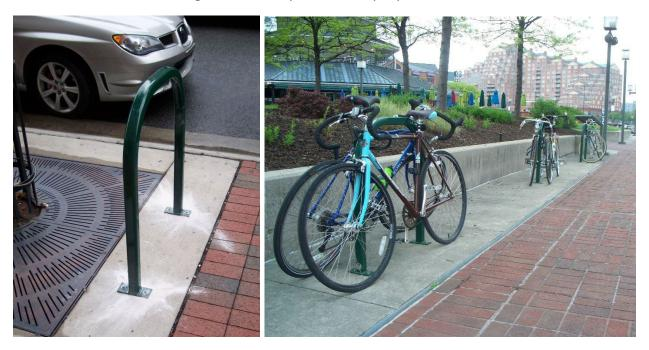
Racks should be stainless steel and utilize surface flange mounting techniques.
