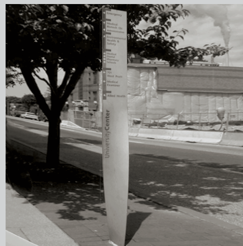
Utilizing the Pohlson light fixture for these directional signs eliminates many of the previous custom signs and eliminates costly brick "inlay" foundations.
