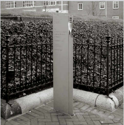
A granite plinth on the new sign eliminates the costly custom brick inlaid foundation that was used on the previous sign.
