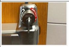
This lecture hall style lock is placed on doors with a push bar. The lock includes instructions so your which way to turn the thumb turn to ensure the door is locked. In this photo, the thumb turn would be turned counterclockwise to lock the door and would be turned clockwise to unlock the door.
