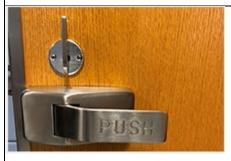
The is like a standard door lock and can be used by turning the thumb turn towards the door frame to lock the door (in this photo, the thumb turn would be turned to the left/counterclockwise.) The thumb turn can be turned away from the door frame to unlock the door (in this photo, the thumb turn would be turned to the right/clockwise.)
